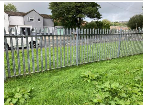
Photograph 22: Example of palisade fencing that surrounds most of the Site.
