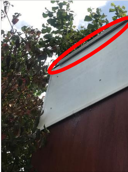
Photograph 36: A gap under the metal roof in the northeast corner of Building 3 with Low suitability to support roosting bats (Figure 1: F3a).
