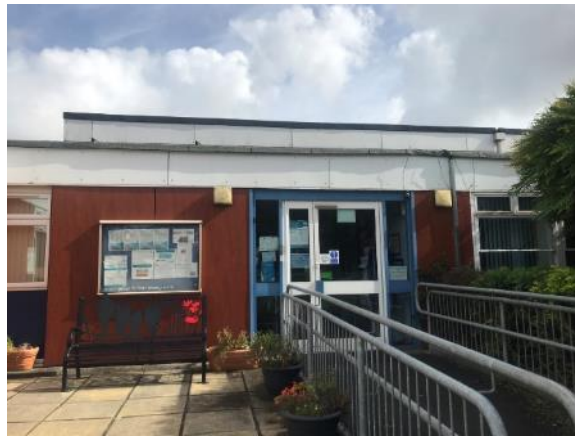
Photograph 29: Building 9 in front and Building 10 behind.
