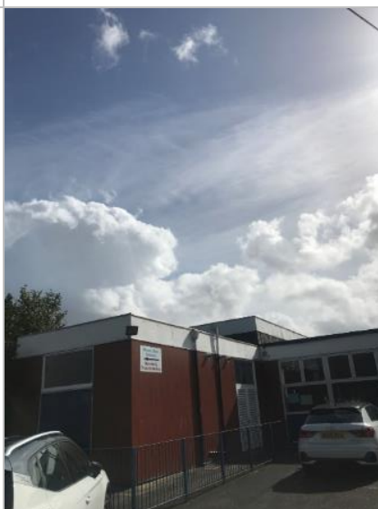
Photograph 24: Building 2 to the right, Building 3 to the left, and Building 4 behind.
