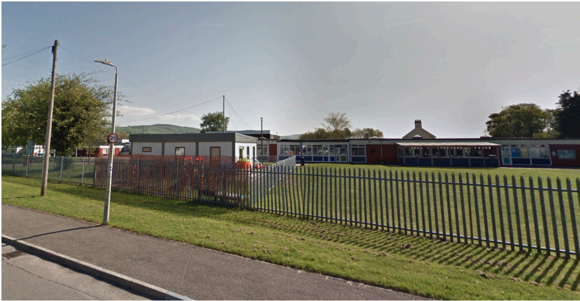
Figure 2: Street View of the site from Caenant Road
