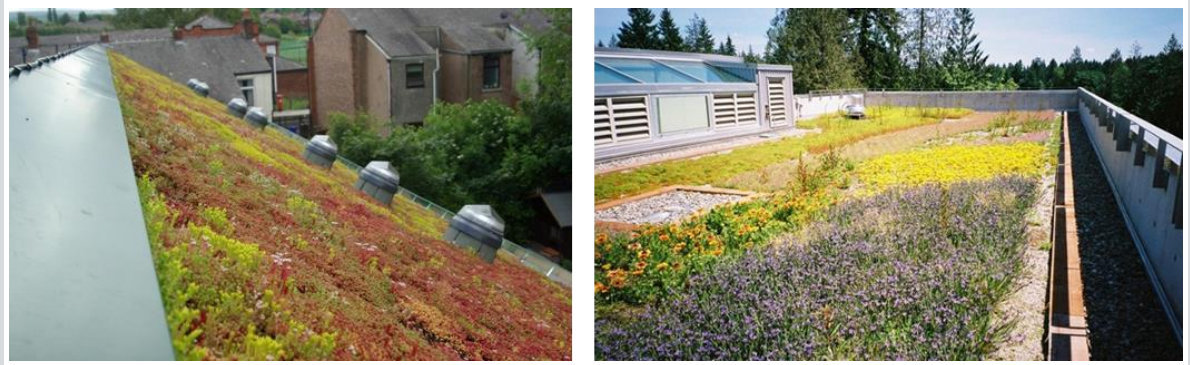
Figure 7. Typical Green Roof Planting
