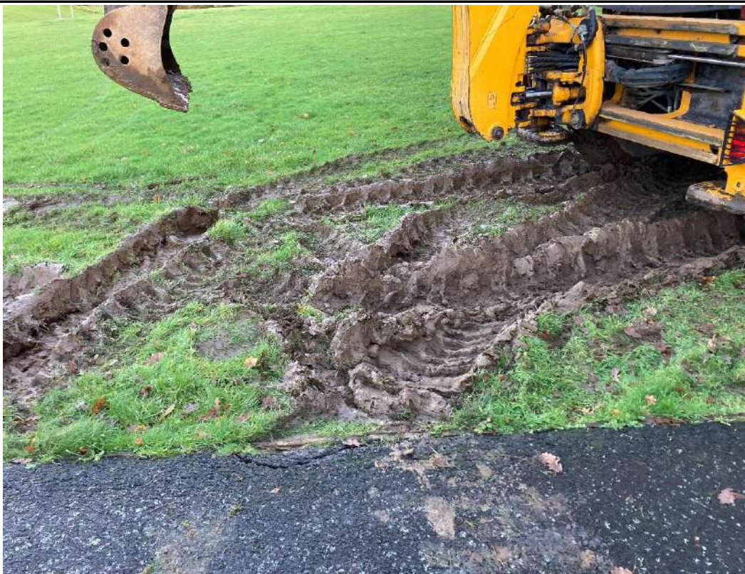
Plate 71 Image of ground disturbance as a result of wet ground during site works
