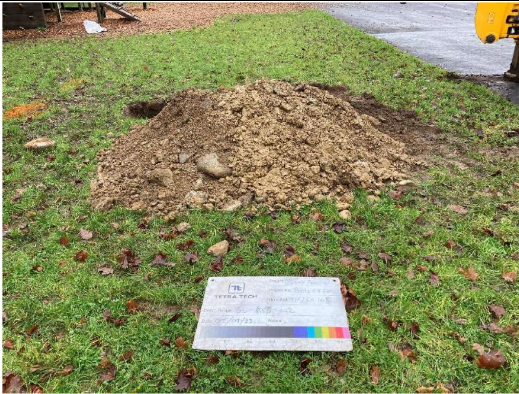
Plate 61 Trial Pit excavation at TP06 location
