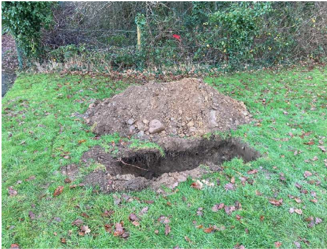
Plate 47 Trial Pit excavation at TP01 location
