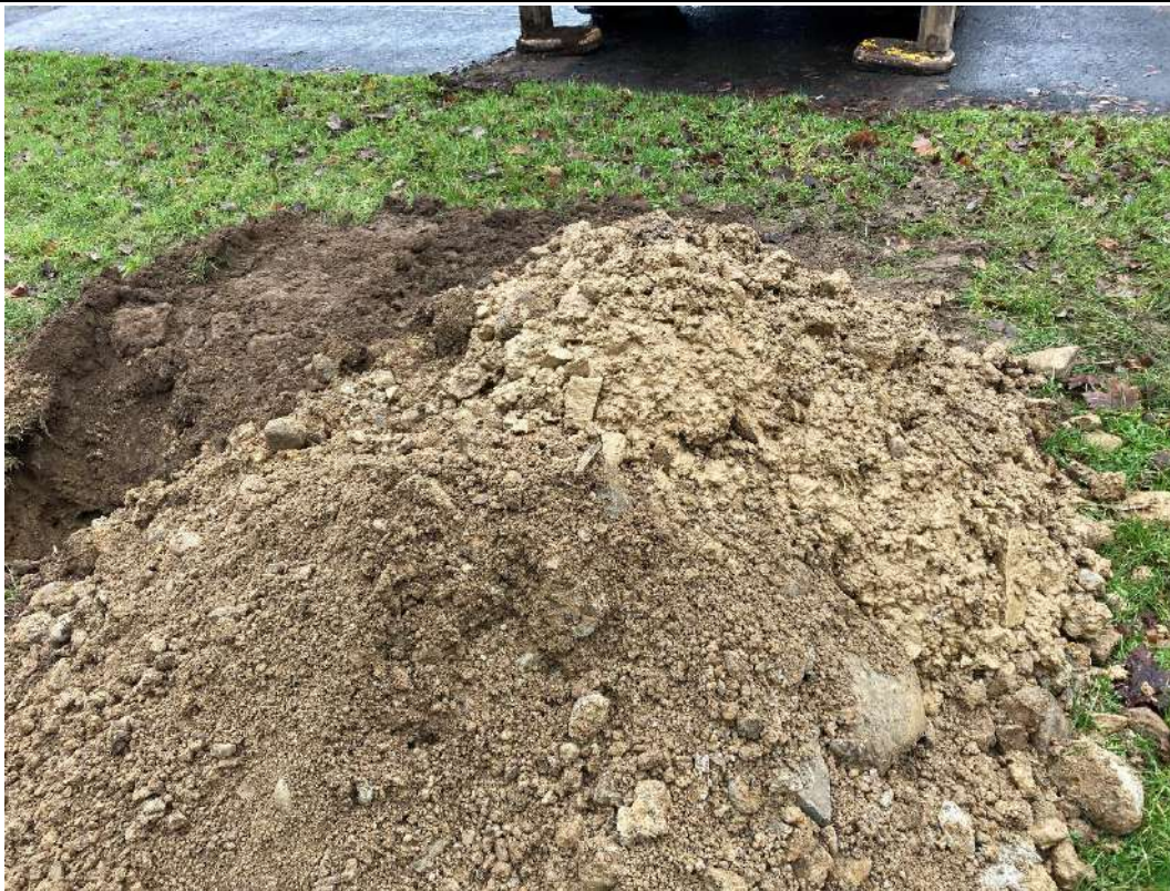
Plate 58 Image of arisings associated with TP06, and positioning of excavator to prevent damage to grass
