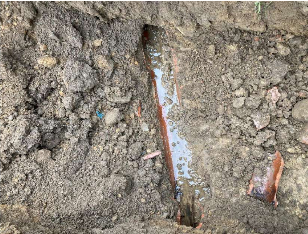
Plate 60 Image of land drain encountered within TP06
