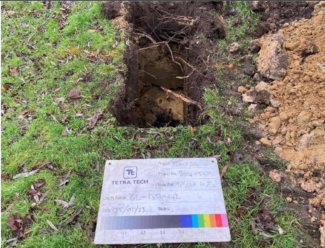
Plate 64 Trial Pit excavation at TP07 location
