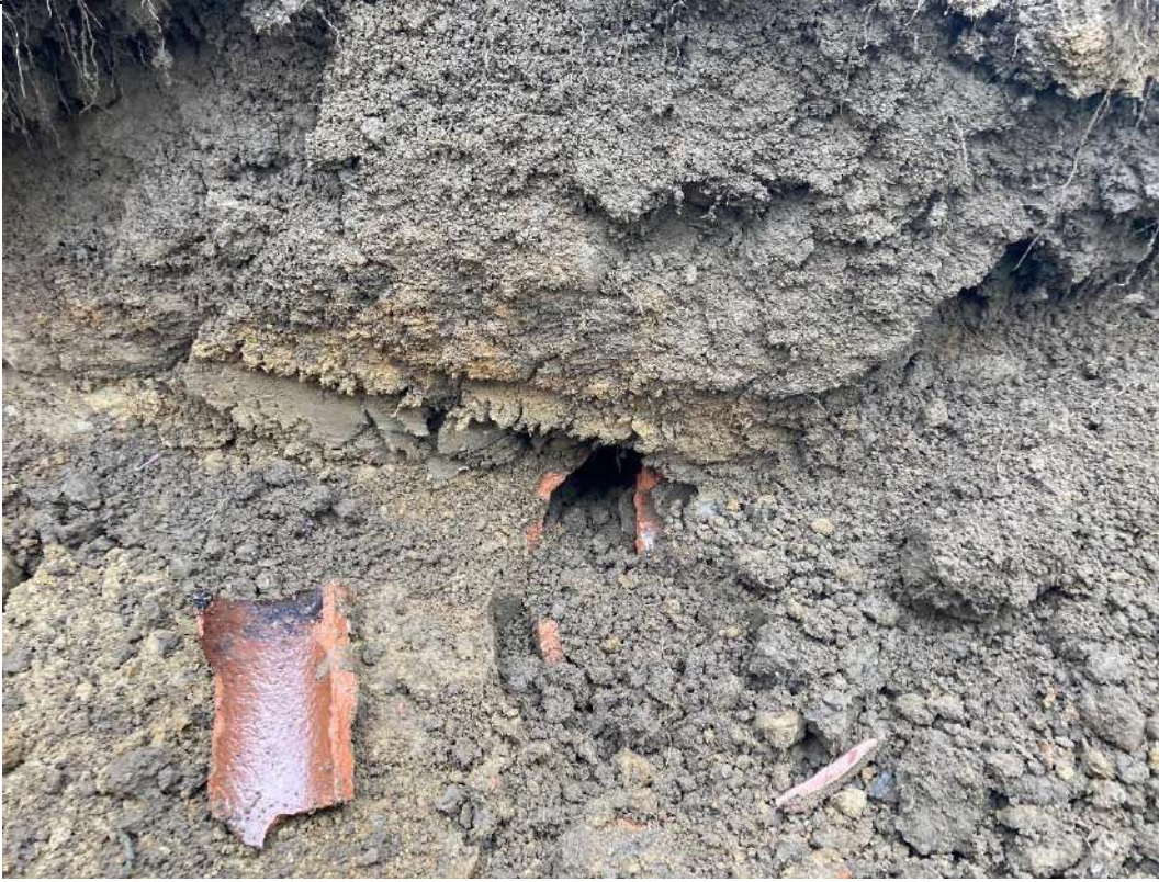
Plate 63 Image of land drain encountered within TP06
