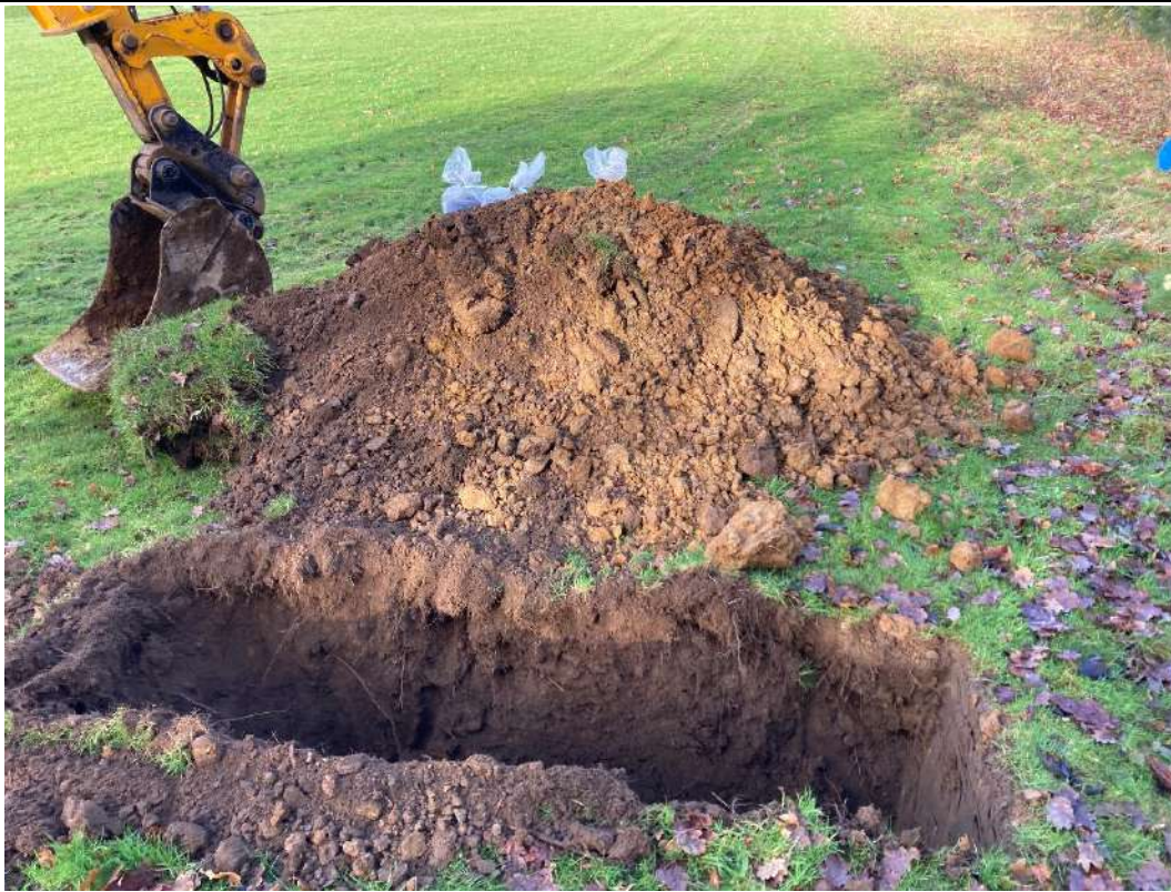
Plate 49 Trial Pit excavation at TP02 location
