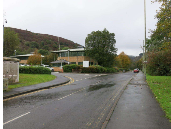
Figure 13: Looking westwards from the north side of the road at the east elevation of Pavilion E showing a belt of introduced shrub and amenity grassland. Large tree is a goat willow.
