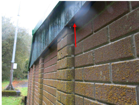
Figure 12.5: Western Garage (south elevation) gaps above brickwork potentially allow bats access to inside of garage.
