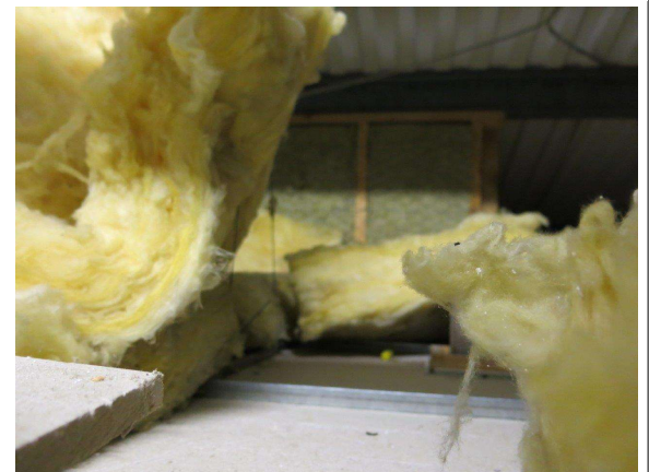
Figure 10.3. Pavilion A roof void showing insulation above suspended ceiling tiles.
