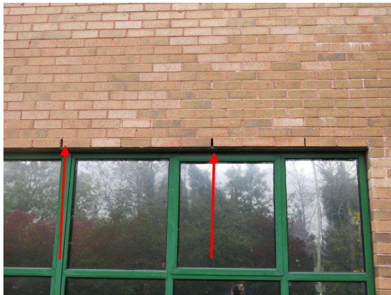
Figure 8.2: Pavilion D – weep hole PRFs above ground-floor window
