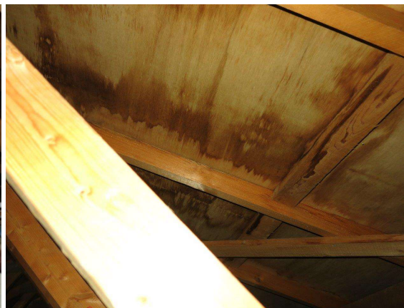
Figure 10.2: Pavilion F roof void showing plywood sarking boards.
