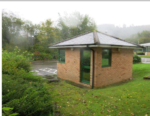
Figure 11.1: Security lodge (north and west elevations).
