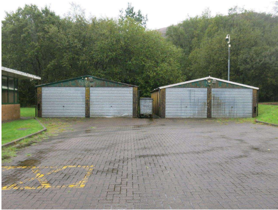
Figure 12.1: The garages (north elevation)
