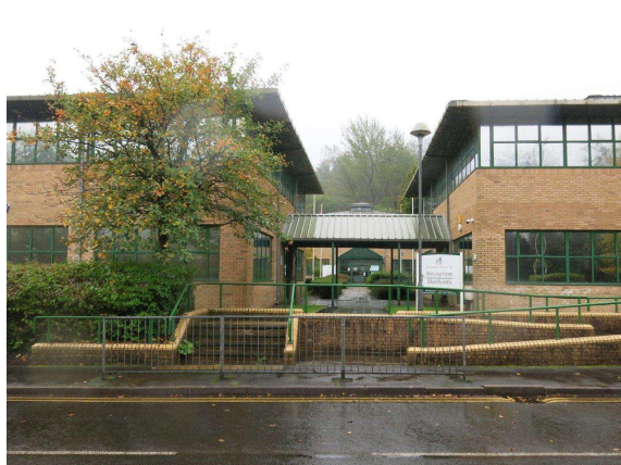
Figure 8.1: Pavilions D & E (north elevation) showing covered walkway between the two.
