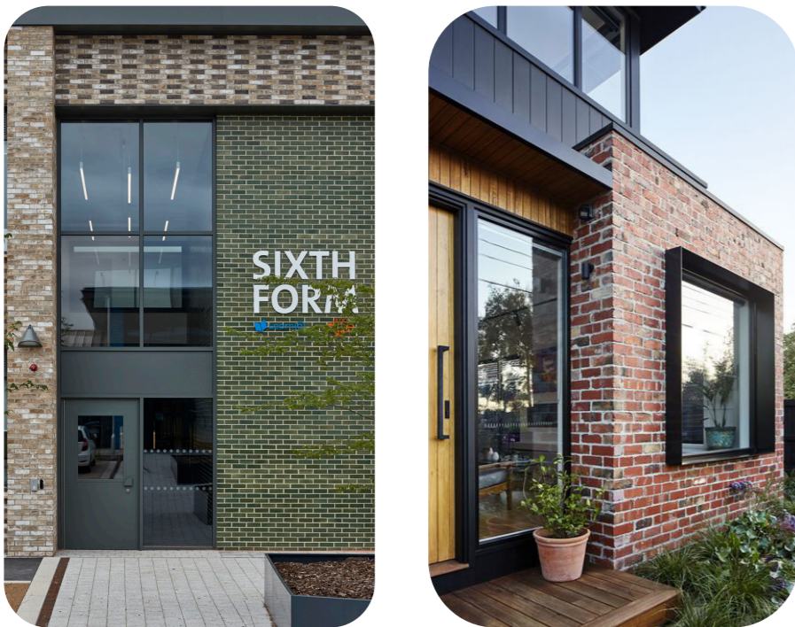
A Recessed entrance and glazed brick
