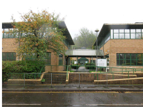
Figure 7.1: Pavilions D & E (north elevation) showing covered walkway between the two.
