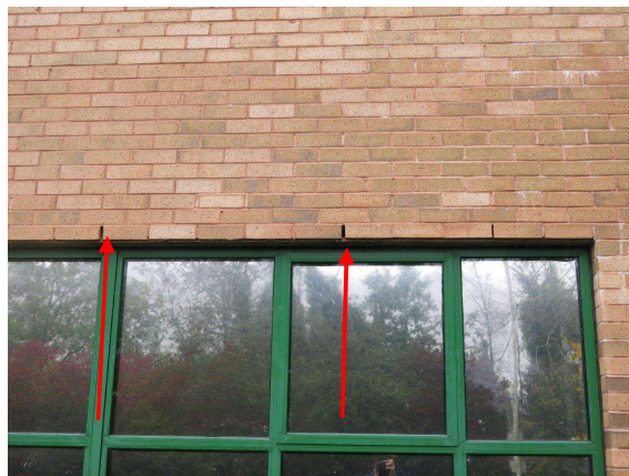
Figure 7.2: Pavilion D – weep hole PRFs above ground-floor window
