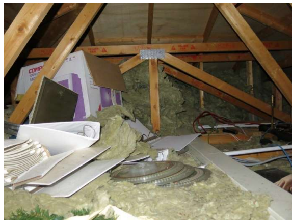
Figure 9.1: Pavilion F roof void – facing north)
