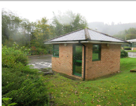
Figure 10.1: Security lodge (north and west elevations).
