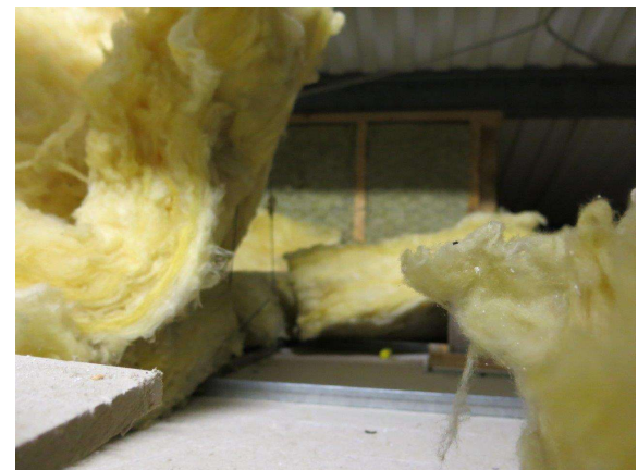
Figure 9.3. Pavilion A roof void showing insulation above suspended ceiling tiles.
