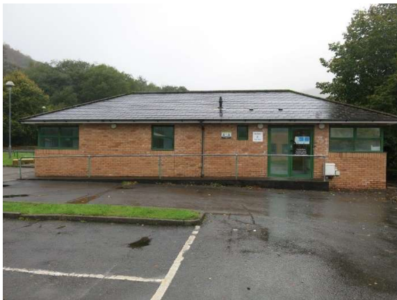
Figure 8.1: Pavilion F ((east elevation)
