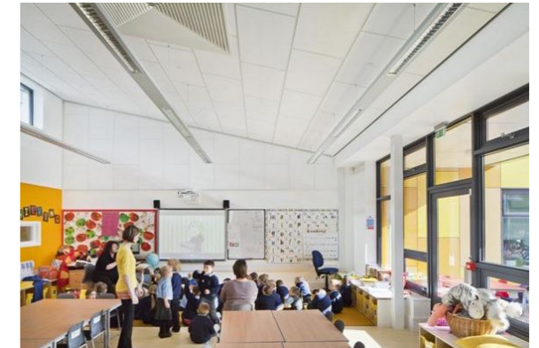
Figure 5: Acoustically absorptive mineral fibre ceilings
