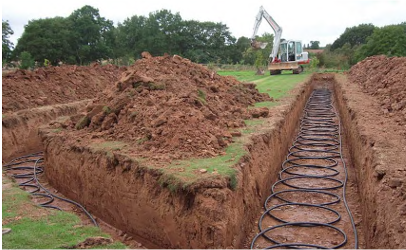
Figure 9 Typical horizontal ground loop
