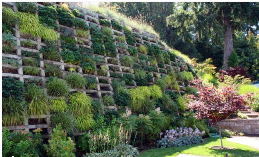
Figure 11 - Example of crib retaining wall
