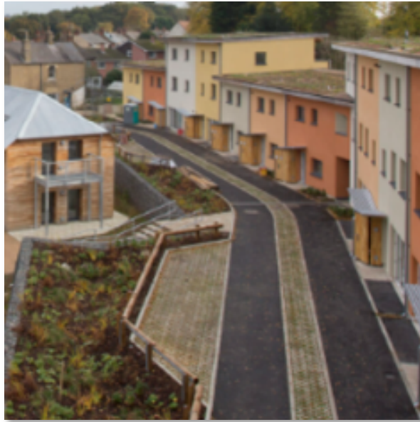
Figure 8 - Example of grasscrete central strip road
