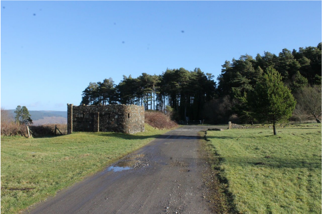
Image EDP A1.6: View to the east of the scheduled monument illustrating the stone walls that define the entrance to the estate and trees of Pelena Forest beyond.
