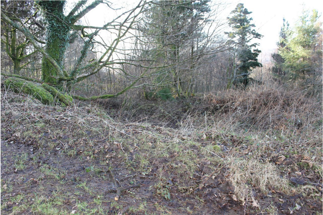
Image EDP A1.20: One of the pits located to the south of Cefn Mawr Colliery possibly reflecting the collapse of underground workings.
