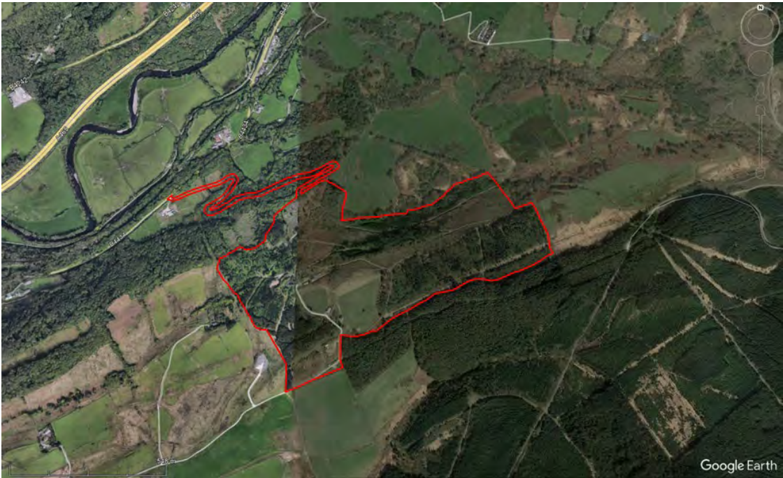
Image EDP 2.1: Birds eye view of the site (Image source: Google Earth, March 2024). Approximate site boundary added by EDP in red.
