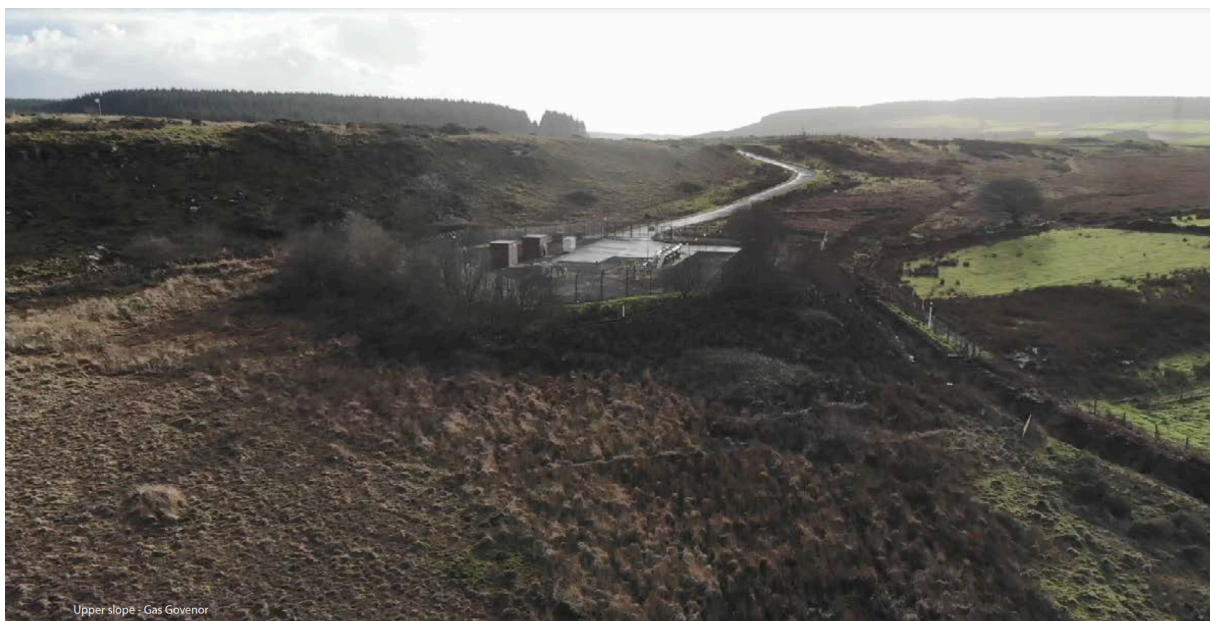
Figure 6: Photograph of the site's upper slope with Gas Governor.
