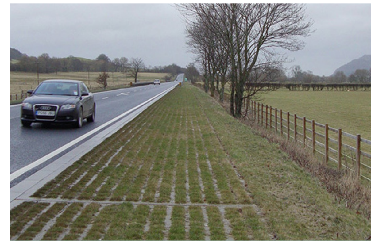
Parking 1A - Grass grate parking: A discrete and natural looking parking surface that can be applied at road edges.
