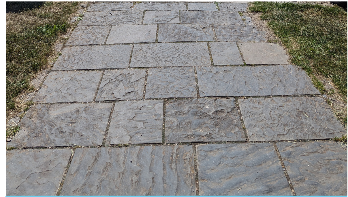
Public Realm 3A - Stone Paving: A natural coloured and textured stone surface material for pathways. Natural stone paving provides a high quality and unifying material in the public spaces of the village.
