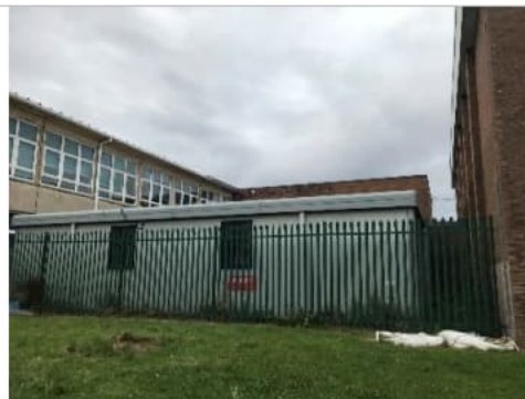
Photograph 2: Building elevation B2b surveyor vantage point.
