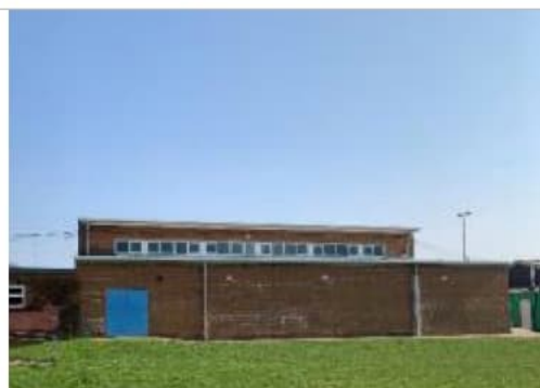
Photograph 4: Building elevation B2d surveyor vantage point.
