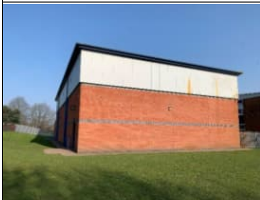
Photograph 5: Building 1 in the centre of the Site. Photo from Wardell Armstrong (2022) 3 .
