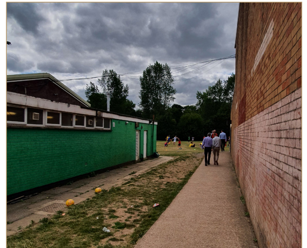
7 - View from existing hard play area (alternative SRB approach)
