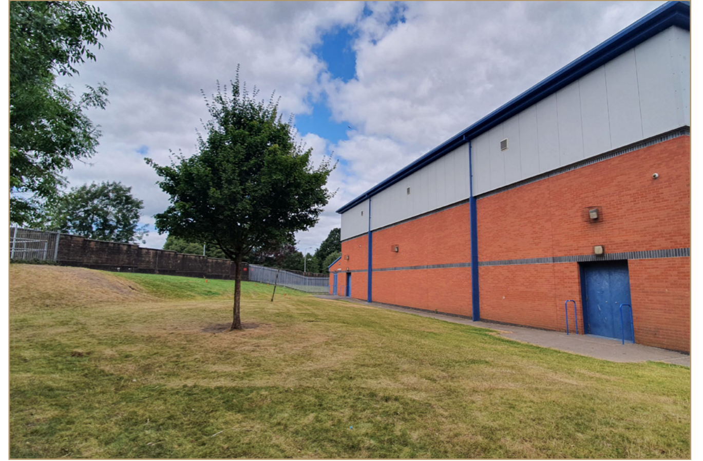
2 - View from the south (proposed location for external M&E and SRB hard-play)
