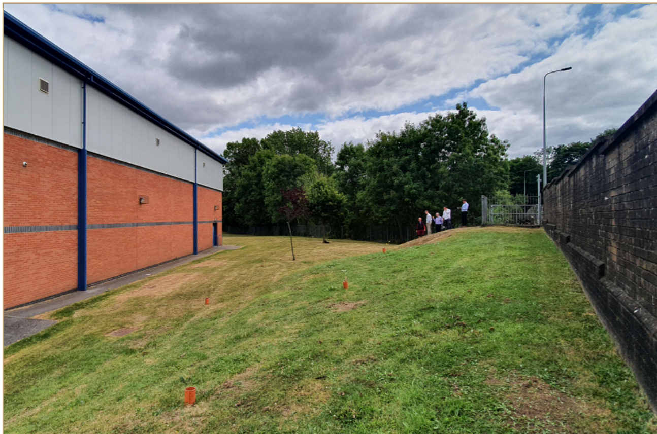
3 - View from the north of site (proposed location for external M&E and SRB hard-play)
