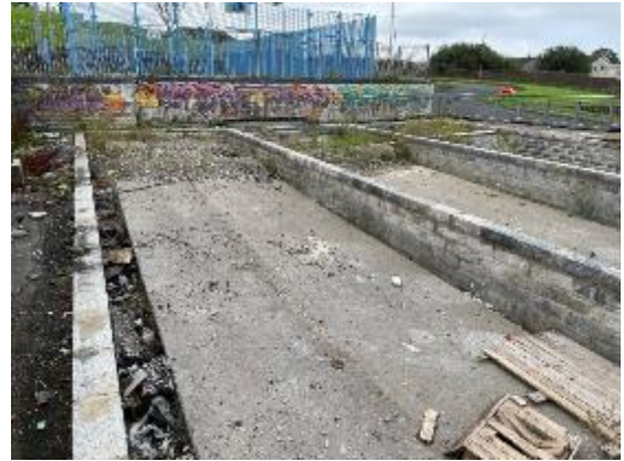
Photograph 4. Site of former building.
