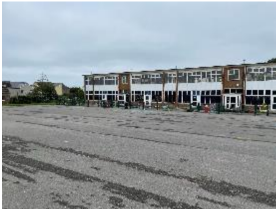
Photograph 3. Building B4 that is proposed for demolition.
