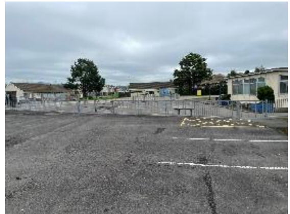
Photograph 4. Areas of hardstanding around school buildings.
