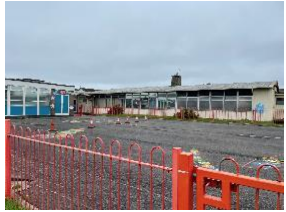
Photograph 2. Building B1 that is proposed for demolition.
