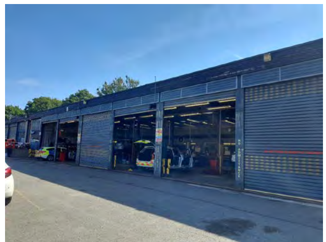
Photo 29. The western elevation of the workshop.
