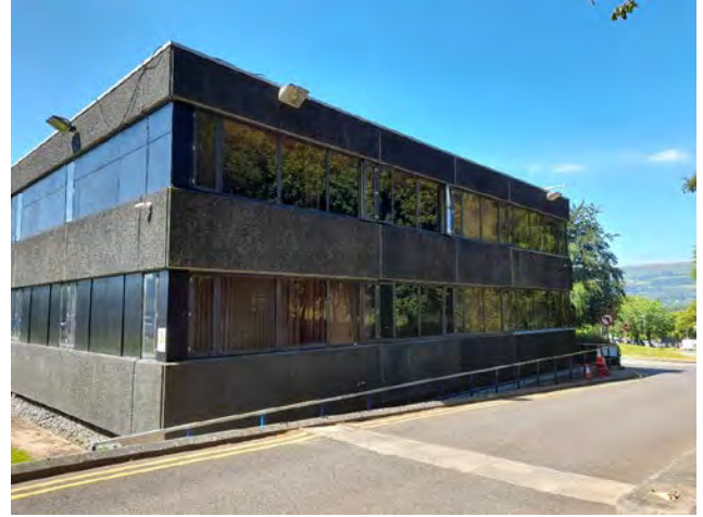
Photo 15. The northern elevation of the administration building.
