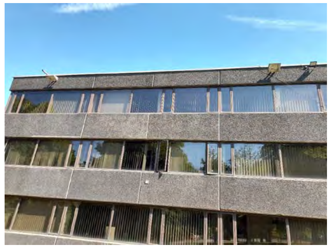
Photo 23. The southern elevation of the amenities building.
