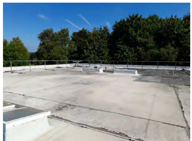
Photo 19. The roof of the administration building.
