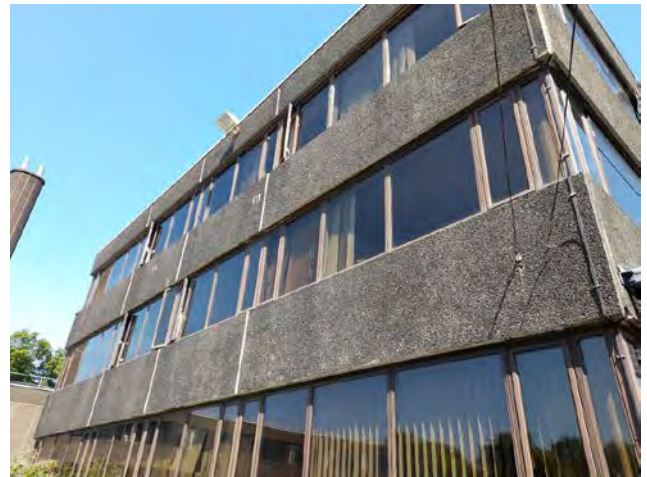
Photo 17. The southern elevation of the administration building.
