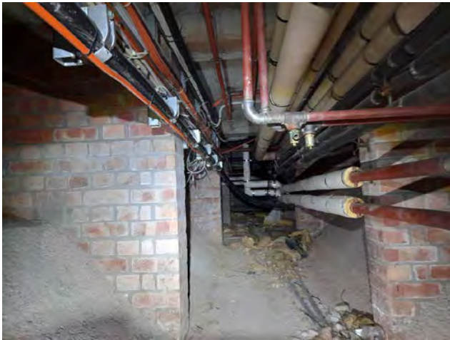
Photo 20. The basement of the administration building.
