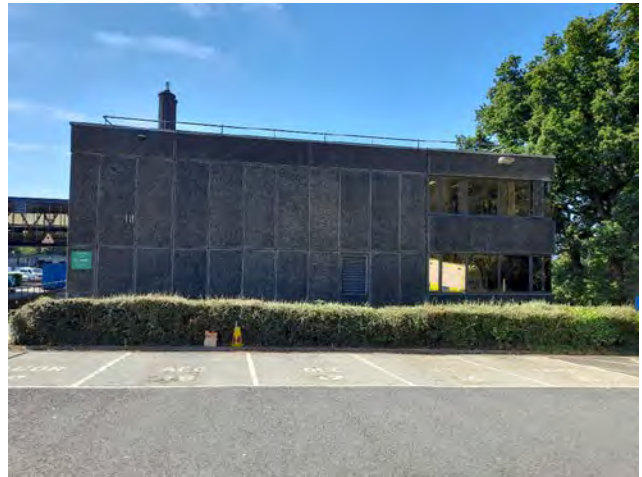
Photo 21. The northern elevation of the amenities building.
