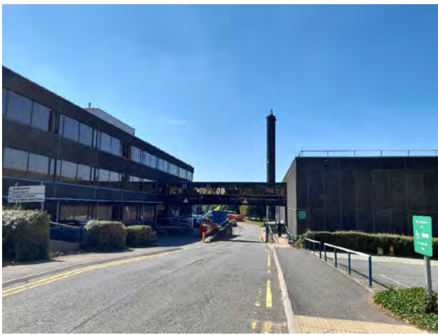
Photo 22. The eastern elevation of the amenities building.
