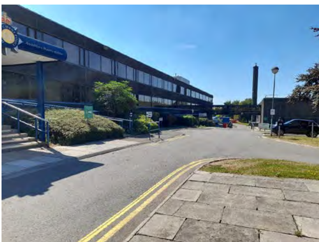
Photo 18. The western elevation of the administration building.
