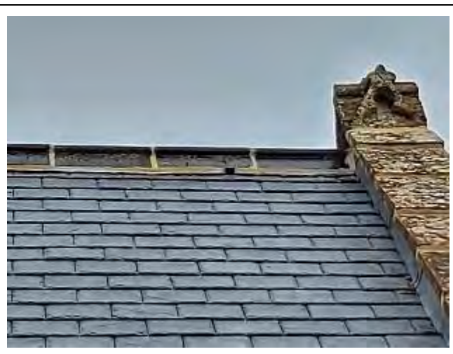
Photo 41. An example of a created access feature suitable for various species of bat within a wet ridgeline.
