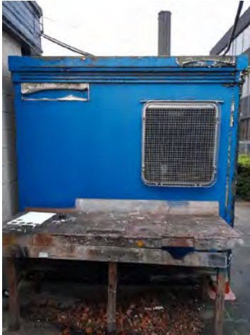
Photo 32. The eastern elevation of one of the temporary buildings located in the eastern section of the site.
