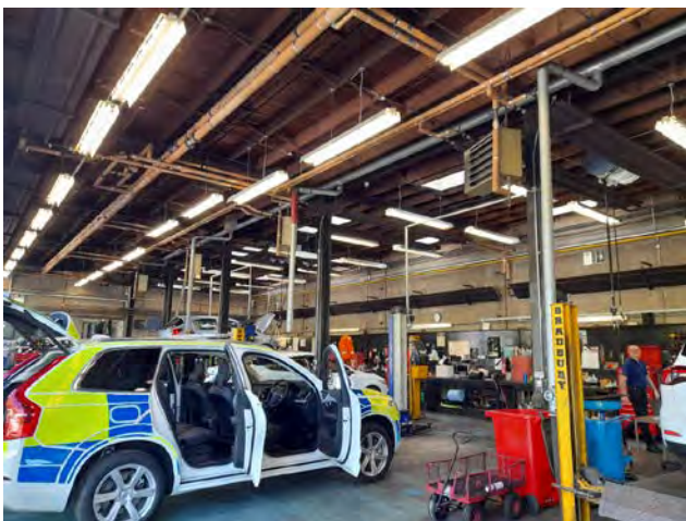
Photo 30. The internal area of the workshop.
