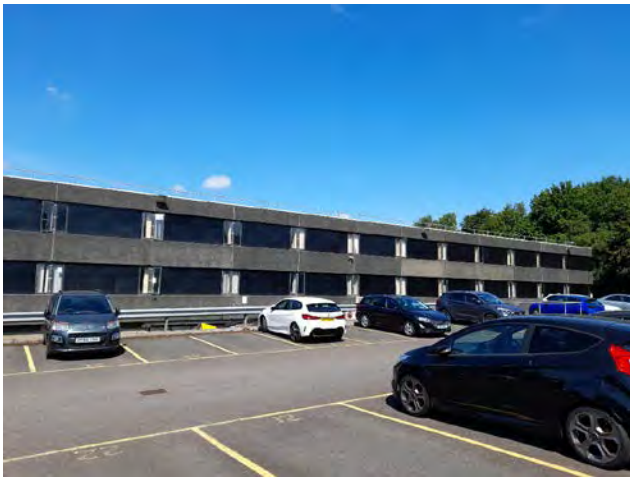
Photo 16. The eastern elevation of the administration building.
