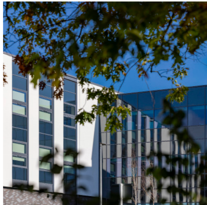
Exeter Police Station A custody suite and associated office space
