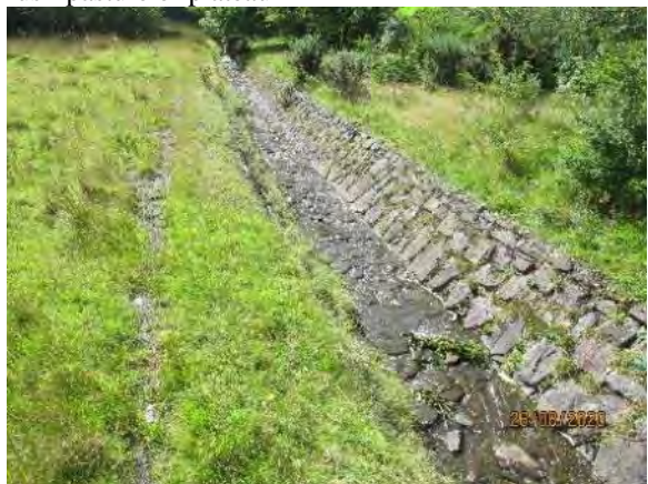
Stone-lined watercourse, typical of site
