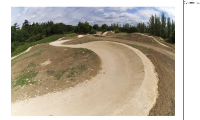
Throughout the radius of a berm the camber of the tread increases until it is near vertical at its top 500 - 2500mm 45° Batter ground level
