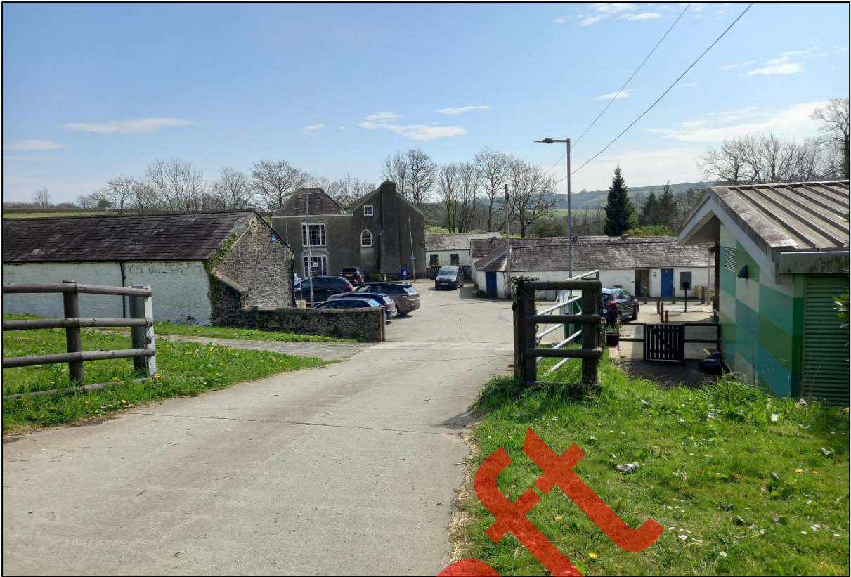
Plate 1: View south-south-east from the South Campus entrance towards Pibwr Lwyd Farmhouse (LB LB9733).
