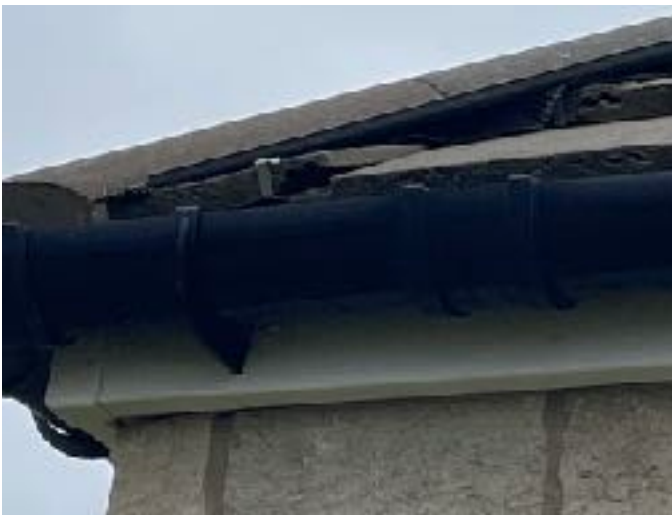
Photograph 9. Electrical building with lifted roof tiles on north and south elevations.
