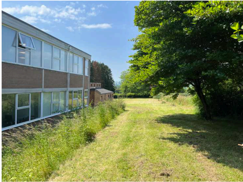
Existing buildings and landscape on the western part of the site.
