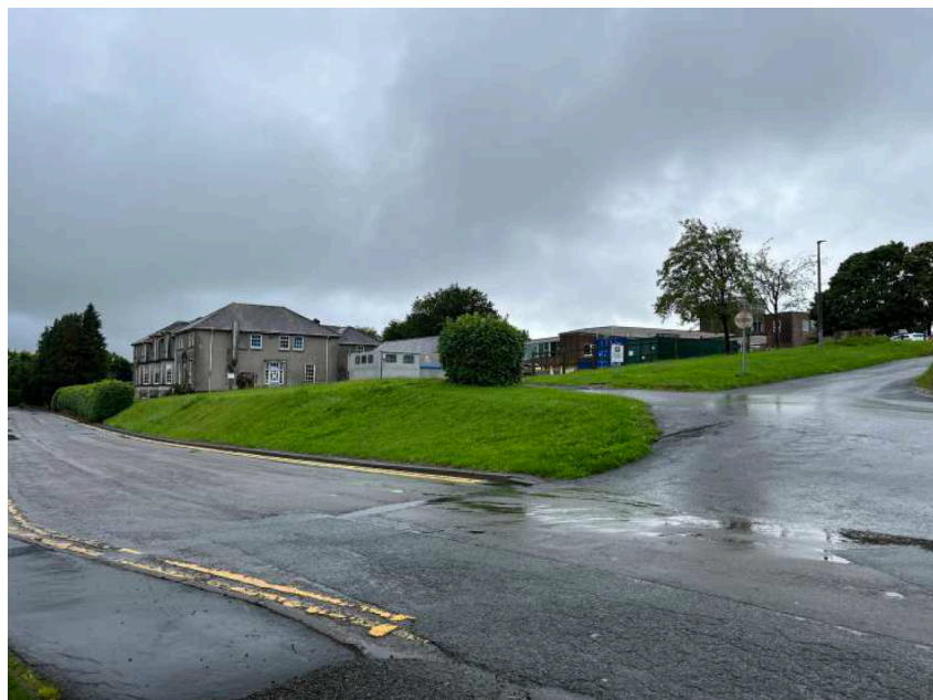
View of existing college buildings and access road from Pibwrlwyd Lane.
