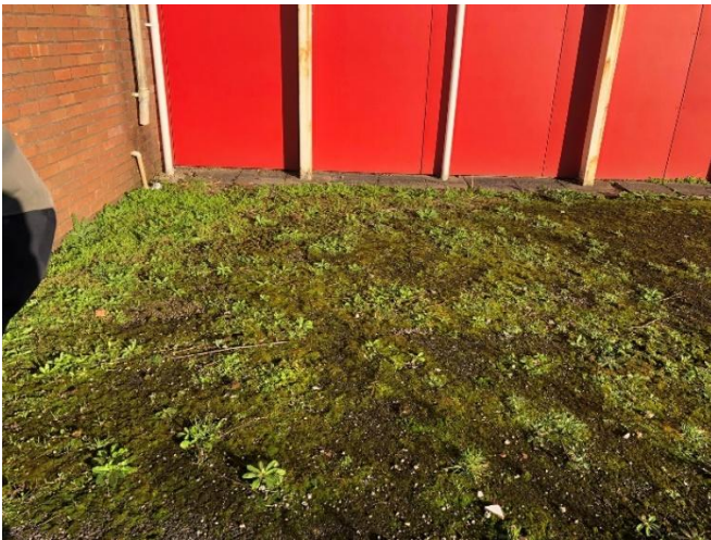
Figure 5- short mossy area within the hardstanding.
