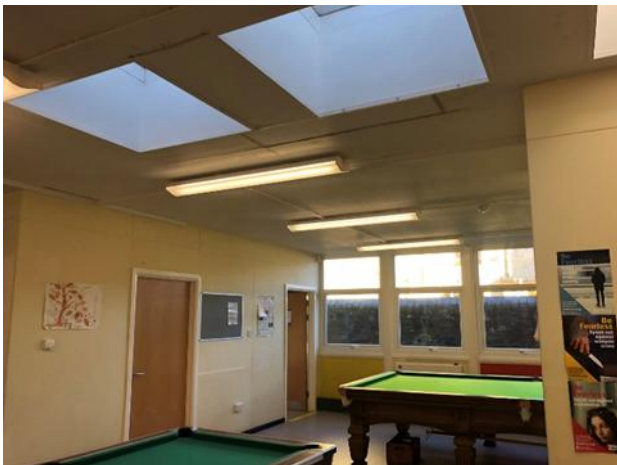
Figure 11- central room of the community centre.
