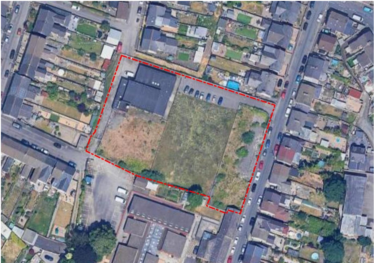
Figure 1- Aerial image of the site (red line shows the site boundary). Image used under licence (©2024 Google). Imagery date 13/11/2024.
