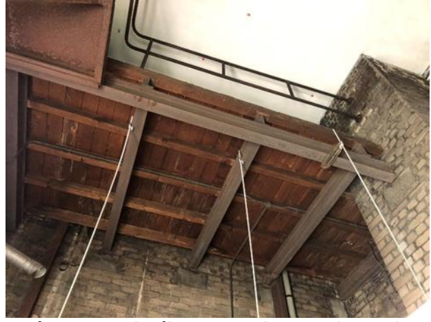
Figure 10- boiler room located south west of the building.
