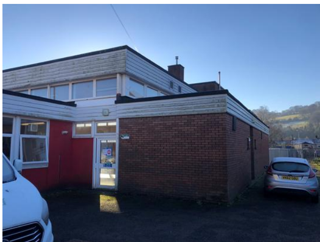
Figure 7- hardstanding and building north-west elevation.
