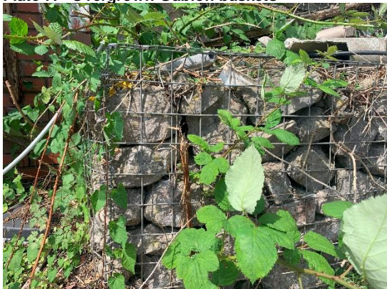
Plate 7: Overgrown Gabion baskets
