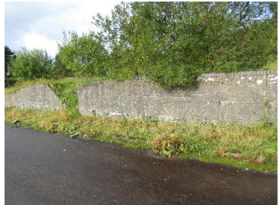
Figure 2.4: Collapsing Retaining wall in north east of the site.
