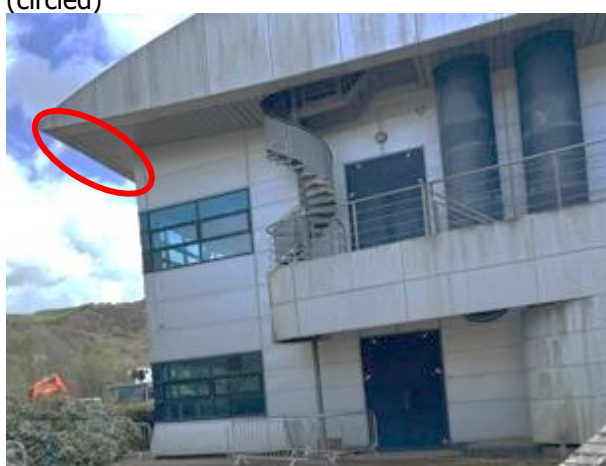
Photo 15: Example of raised capping of soffit box (circled)
