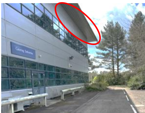
Photo 14: Example of raised soffit (circled)
