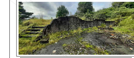
IMAGE 3: RETAINING WALL IN THE PREVIOUSLY DEMOLISHED AREA OF THE SITE
