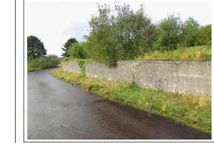
IMAGE 2: RETAINING WALL IN THE NORTH-EAST OF THE SITE IN POOR CONDITION, WITH INSUFFICIENT DRAINAGE CAUSING BLOCK WASHOUT.
