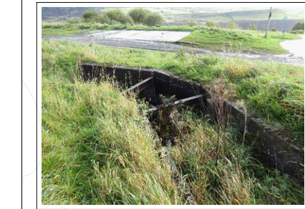
IMAGE 1: EXISTING HEAVY DUTY HEADWALL
